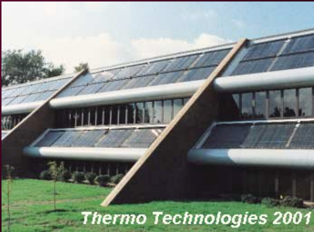
Figure: Installation at Kalamazoo D.O.T.
