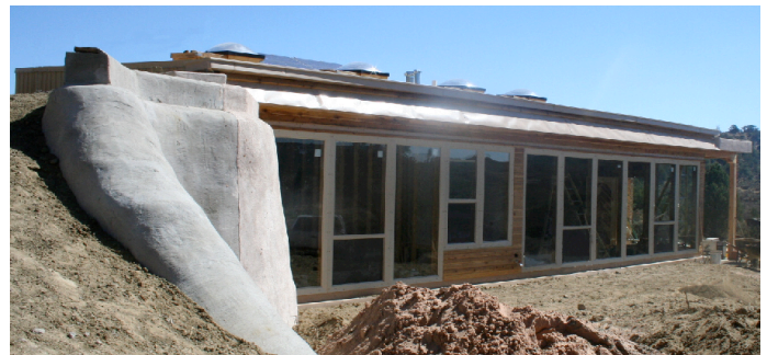
Fig. 1 One bedroom earthship located in Gamerco, New Mexico
