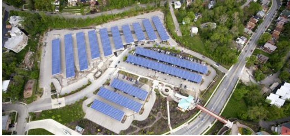
Figure 2: Cincinnati Zoo Solar PV Parking Canopy
