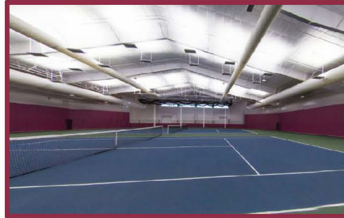
Interior View of Huizenga Tennis and Track Center
