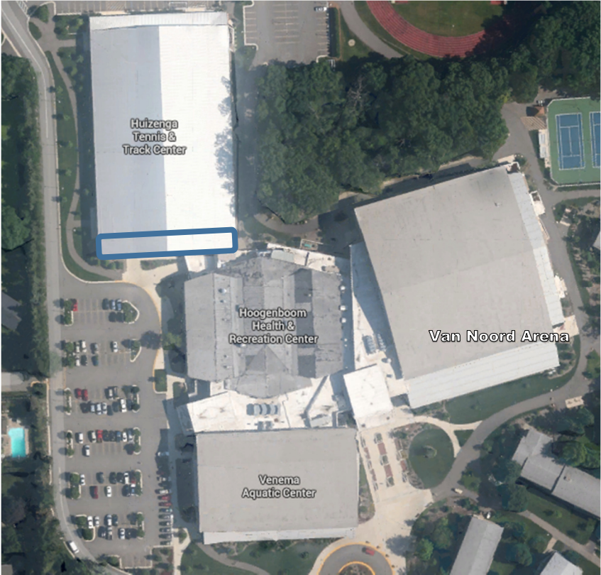
Figure 29: Inverter Location in T&T Utility Room (shown in blue rectangle)
