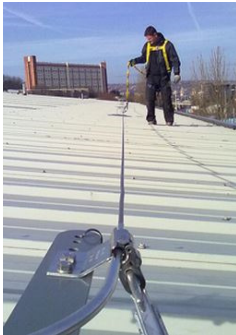
Figure 26: Safety Harness System [12]
